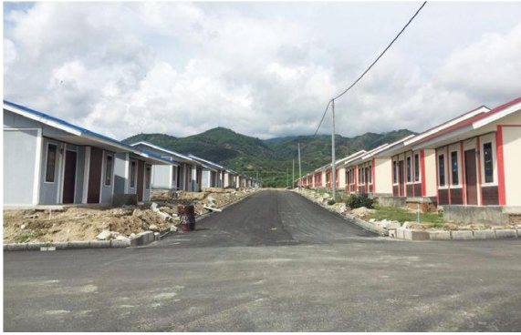
Housing units for ASEAN Village Project, Palu City. Source: ASEAN Coordinating Centre for Humanitarian Assistance on disaster management
